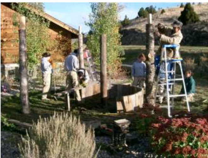
Americorps Volunteers and John Ellingsen building the Arrastra.
