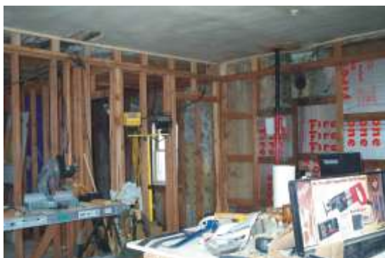
Demolition of modern features reveals historic treatments to walls and ceilings.
